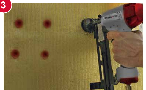
FS9240BC securing insulation layers
