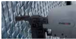
Lath attachment using one-inch TrakFast discs and magnetic probe
